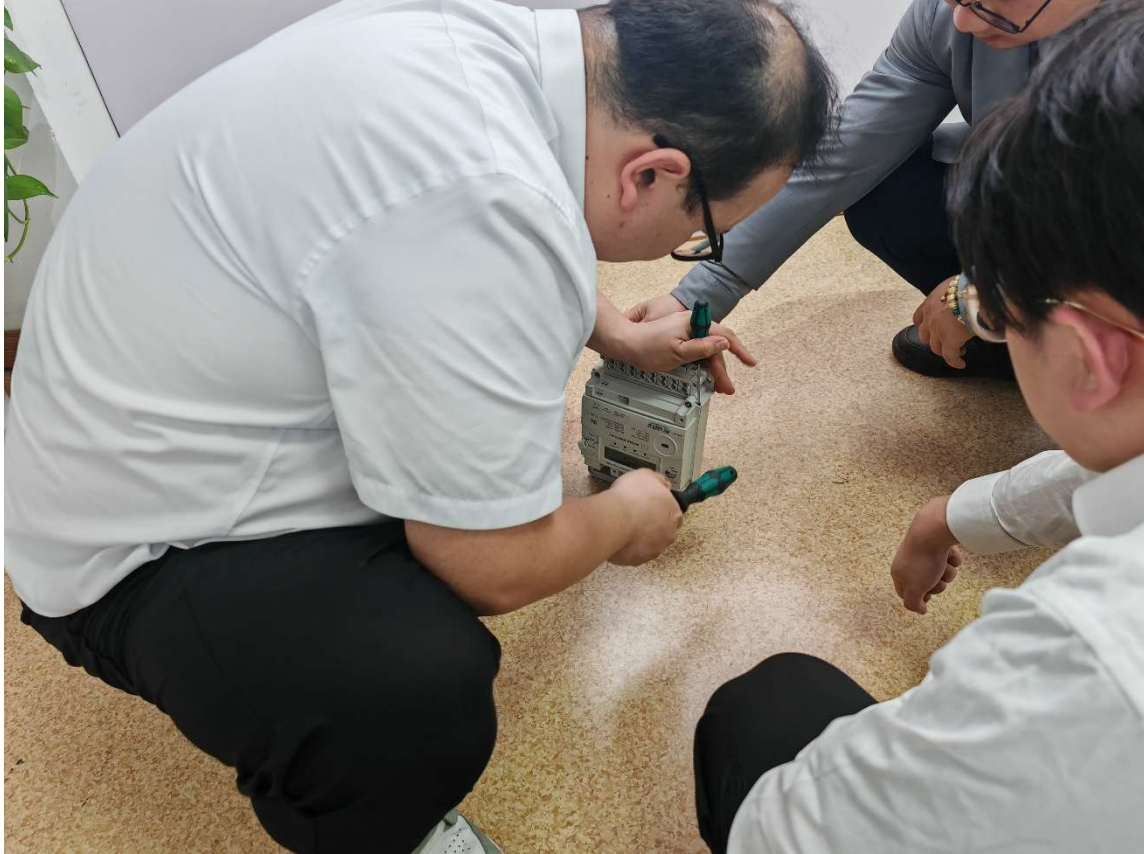
On-Site Disassembly Of The Relay
